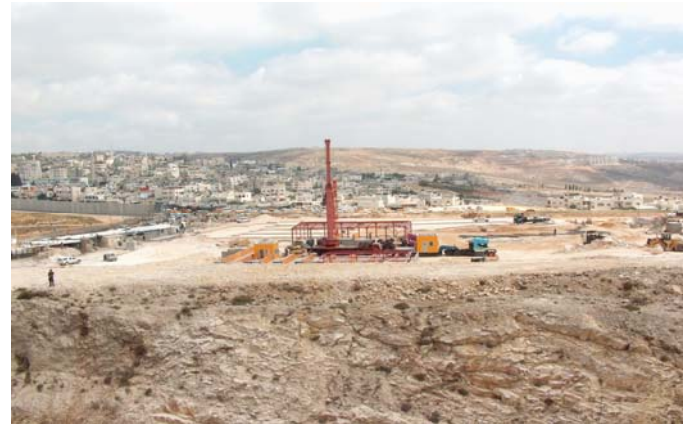
OCHA – Jerusalem FCU – 2005 | Construction work at Qalandiya Checkpoint
